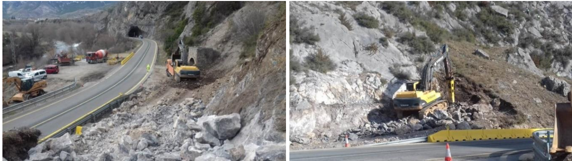
Fig. 4 - Drilling works of the new South tunnel mouth
