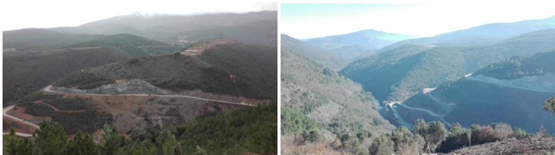
Fig. 3 - Alto Tamega Construction Site overview
